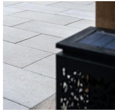
**NEW PAVED AREA MATERIAL - UNILOCK METRO CONCRETE SLAB**
